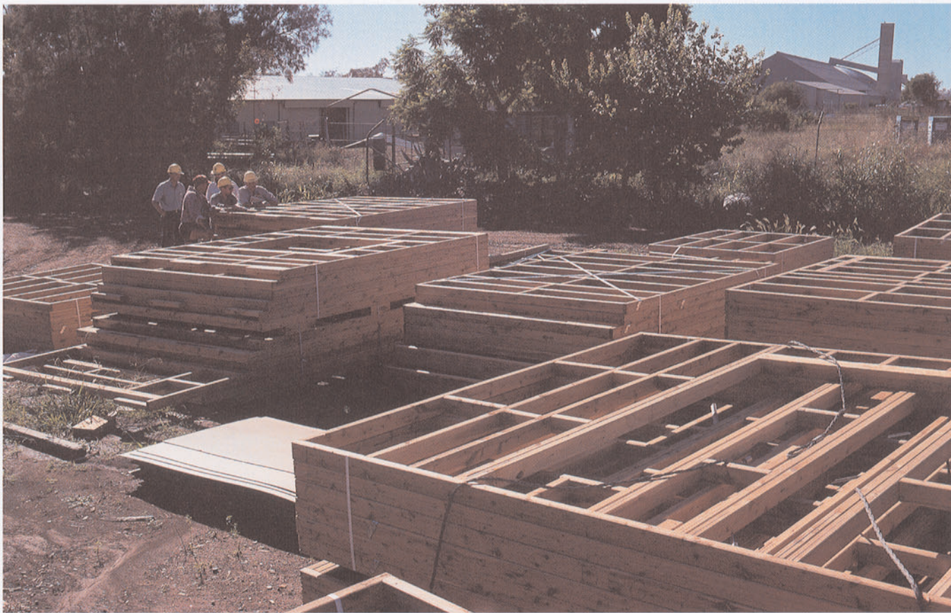
Prefabricated wall frames made from white cypress pine.
