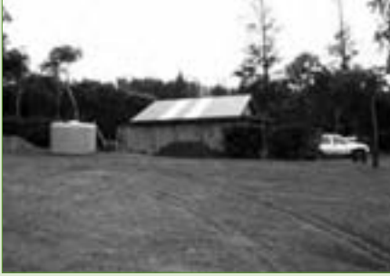
The new amenities are constructed to match the traditional Norfolk Island building style, using locally sourced Norfolk Island pine
