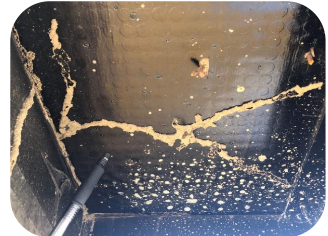
Termite tunnelling underneath shipping container.
