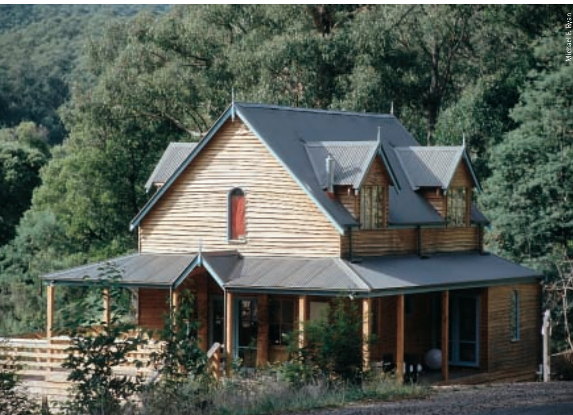
Radially sawn timber weatherboard house
