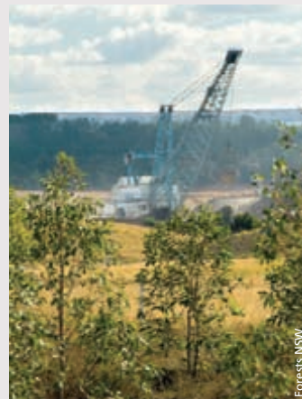
Narama Mine rehabilitation, New South Wales.
