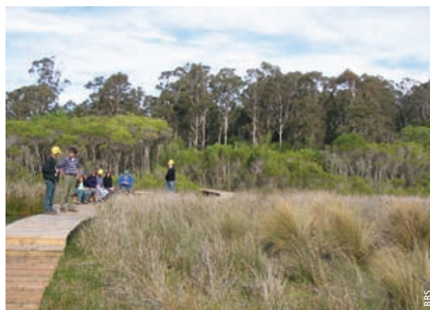
A boardwalk installed to prevent foot traffic from damaging vegetation and soil at a sensitive site.
