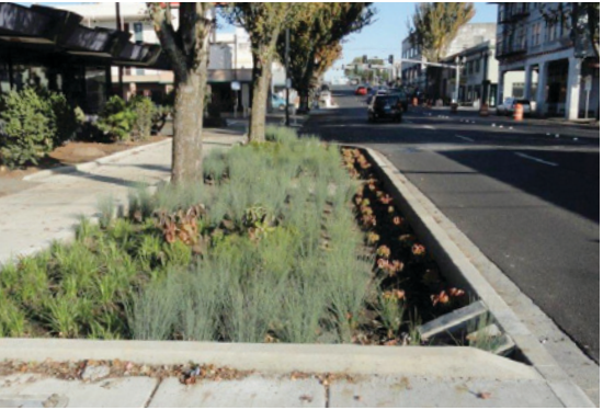
Stormwater WSUD Trench
