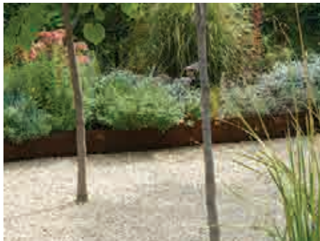
Rusted mild steel bed edging.
