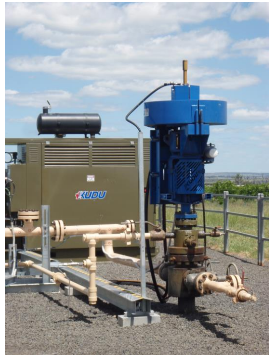
Figure 13 Typical coal seam gas wellhead in Queensland (© Copyright, DSEWPaC 2013; courtesy B. Gray and Origin Energy).
