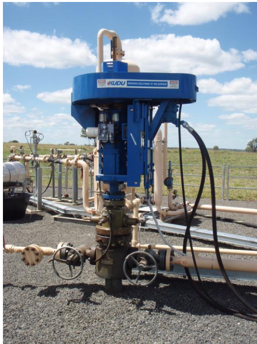
Figure 13 Typical coal seam gas wellhead in Queensland (© Copyright, DSEWPaC 2013; courtesy B. Gray and Origin Energy).
