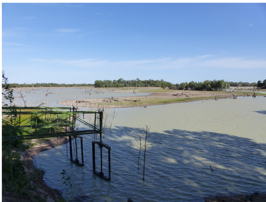
Figure 2-7 Boera Dam with regulator pipes in foreground, western floodplain bywash to the left and main Warrego river flowpath to the right (photo D.Ryder)
