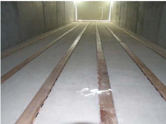
*Inside a composting tunnel with aeration channels*
