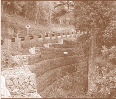
An example of a gabion wall and steep cutaway along Mount Pitt road, minimising plant loss and watershed interruption.
