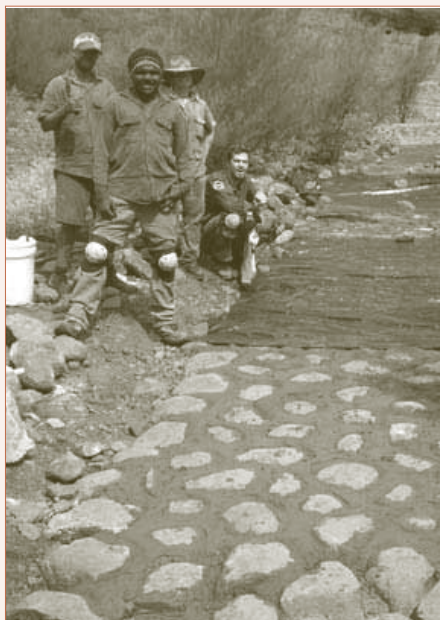
Construction of the hardened surface along the Valley of the Winds track
