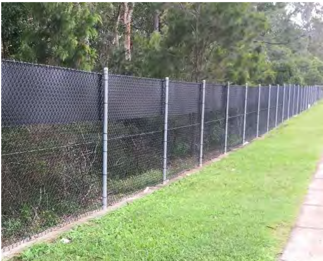
Figure 6: One direction exclusion fencing along northern side of Yawalpah Road (Location 3)
