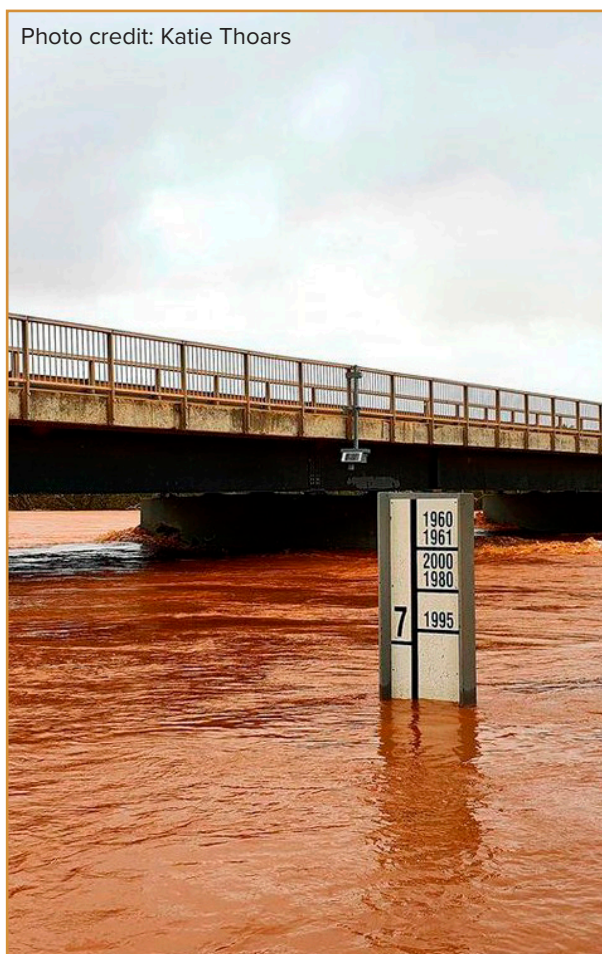
Figure 15: Flood gauge at Nine Mile Bridge on the Gascoyne River showing historic flood levels
