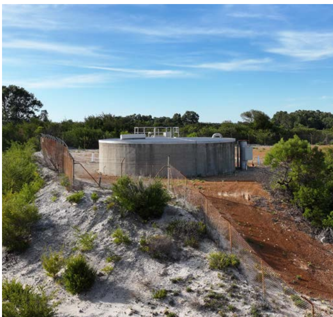
Image: Regional water infrastructure, Esperance
