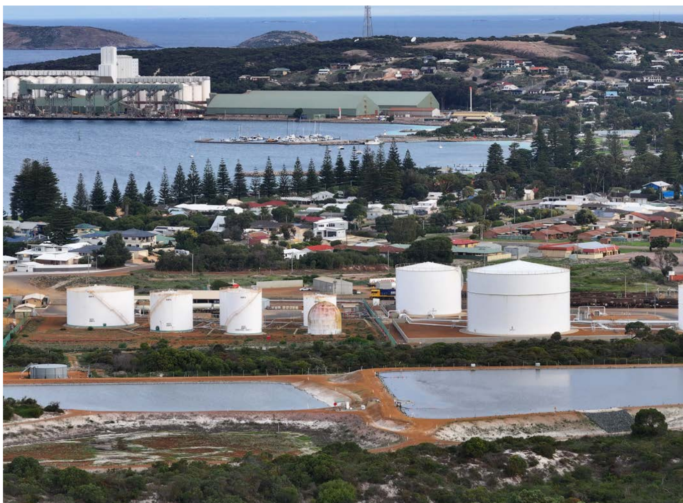
Image: Wastewater Treatment Facility, Esperance
