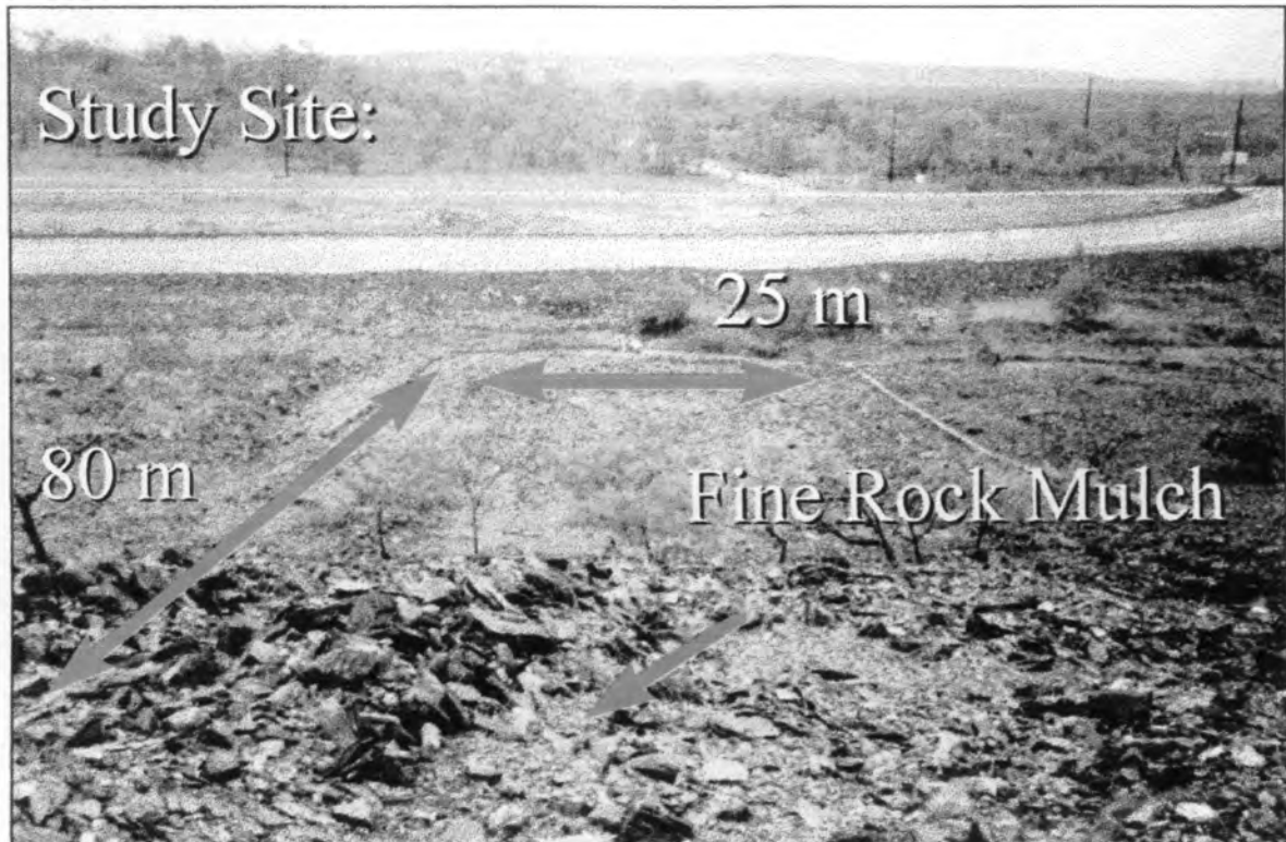
Figure 1.1.4: The batter slopes of the Northern waste rock dump has been exposed for a period of several years. Some natural re-vegetation had occurred, which was not considered to have any impact on the erosion study. It was also noted that relatively fine material has accumulated in the upper surface layers of the study site.
