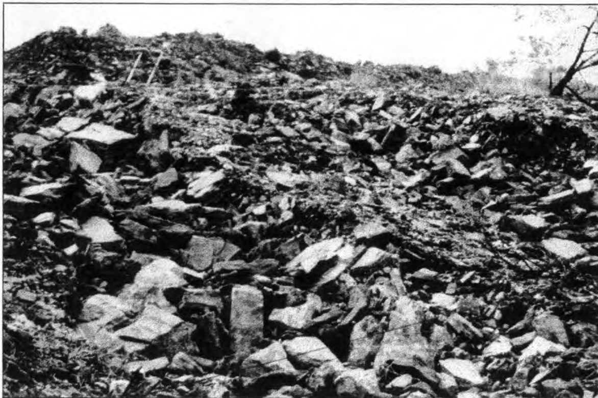
Figure 3.2.9: The profile of the upper section was established by the first major storm event. Complete removal of fine material is evident in this figure and comparison is made to Figure 3.2.8 above.
