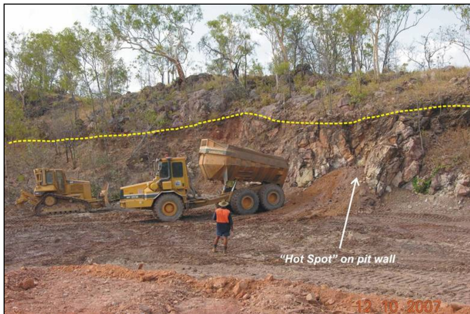
Figure 3 Sleisbeck pit during backfilling (photo: M Fawcett)
