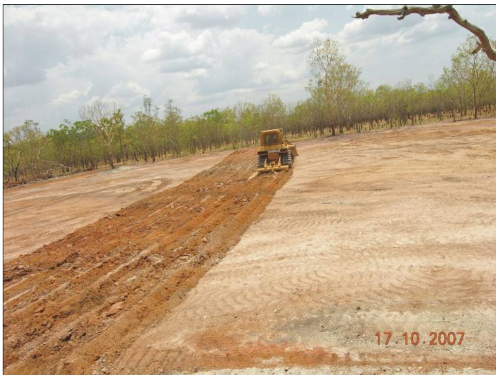
Figure 5 Ripping the footprint of the former truck dumps (photo: M Fawcett)
