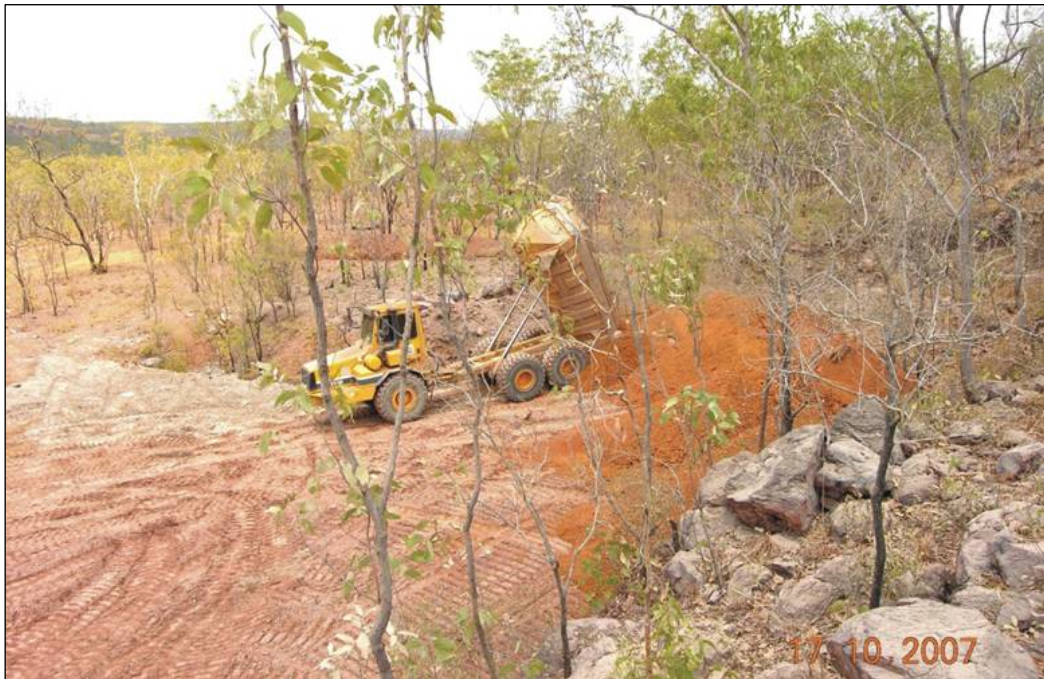
Figure 4 Placing of the low radioactivity cover layer over the pit (photo: M Fawcett)
