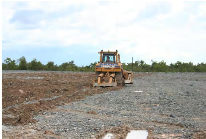
**Figure 3** Ripping the surface of the trial landform. The mounds created by the tynes can be seen as well as the area yet to be ripped.
