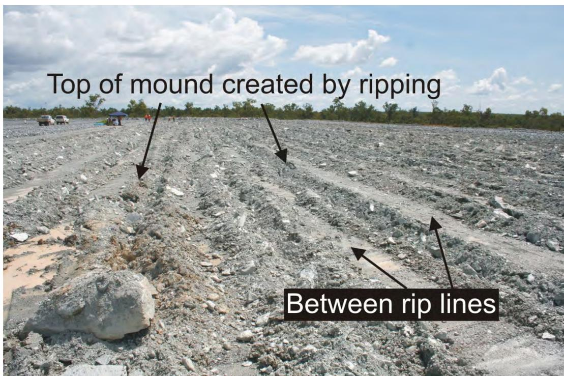
**Figure 6** Shows the top of mounds created by ripping and the areas between the rip lines. A large boulder is also visible in the bottom left of the image.
