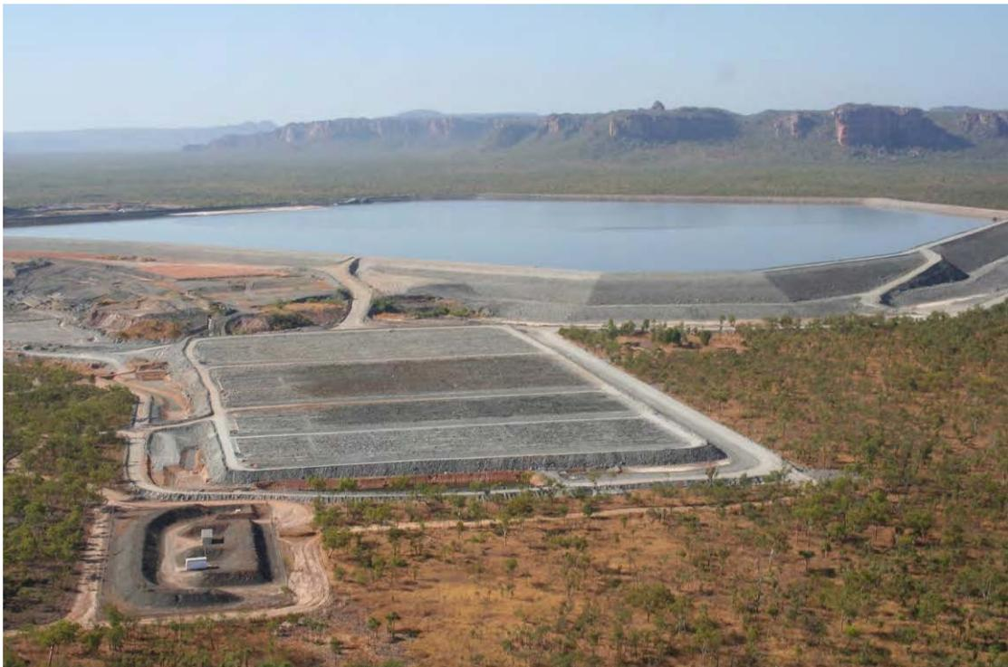
**Figure 1** Aerial view of the completed trial landform located next to the Ranger mine Tailings Storage Facility (taken 28 August 2009 by M Saynor)
