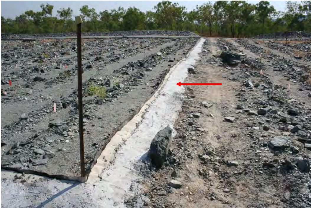
Figure 6 Concrete along the top boundary of EP2 to seal the breach and reinforce the boundary. The red arrow shows where the breach occurred.
