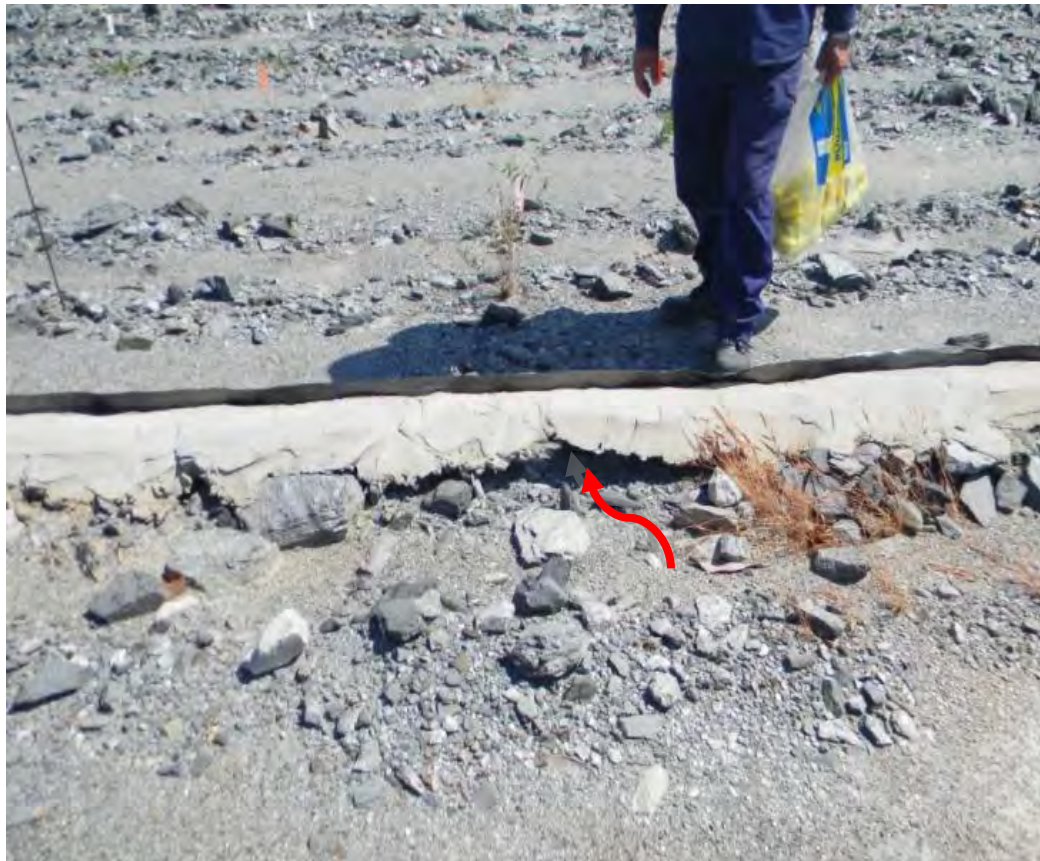
Figure 5 Piping failure under the top boundary of EP2 indicated by arrow.
