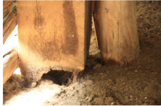
Photo 1 Posts in 'white man's' houses rotted away and needed to be supported using local hard wood shown here.
