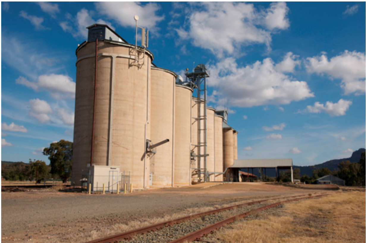
Silos near railway track © Department of Agriculture, Water and the Environment
