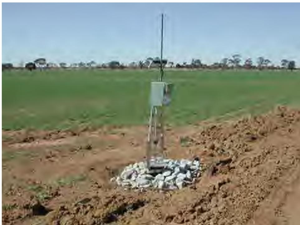
**Figure 8. Telemetry Controlled Riser Outlet (Source: Archards Irrigation)**
