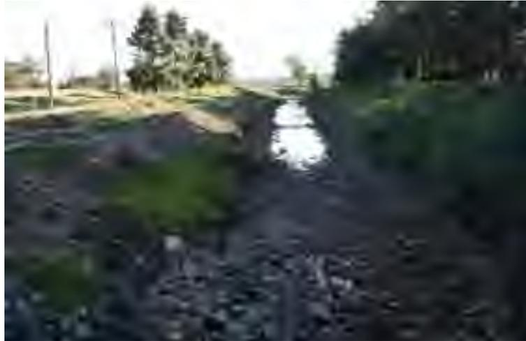
**Figure 2** Main Jemalong supply channel (earthen channel) for the Jemalong Irrigation scheme.
