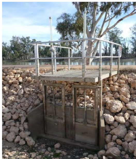
Figure 4.6: Penstock Vertical Winch (Photos: M Harper).
