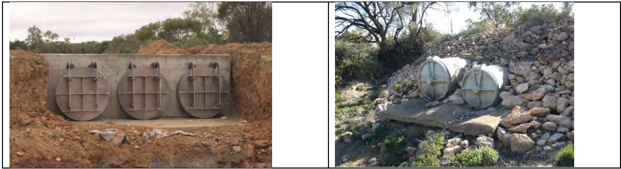
Figure 4.5: Sample of metal and fibreglass hinged flap gates (Photos: B Rampano and M Harper).
