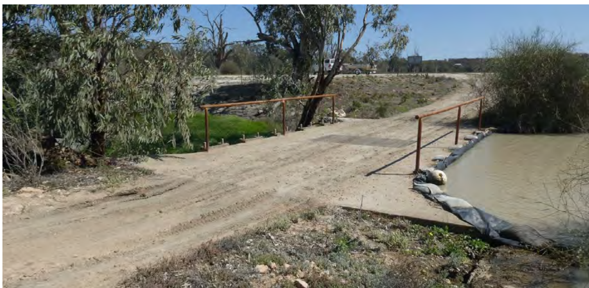
Overland Corner outlet structure - Note the plastic on the wetland side to hold back pumped water. (Photo: by M Harper)
