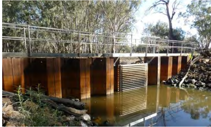
Figure 4.9: Metal Sheet Piling structure fitted with segmented Stop boards. (Photo: M Harper).
