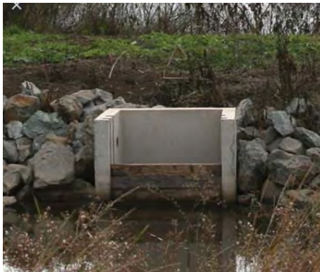
Figure 4.7: Wooden stop logs fitted to a drop board culvert (Photo: M Harper).
