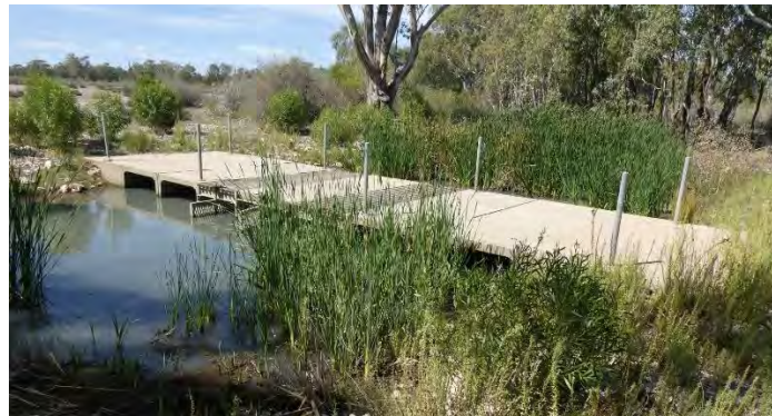
Existing Box Culvert inlet structure which does not hold water
