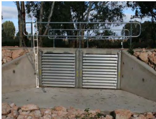
Figure 4.8: Segmented stop boards fitted to a box culvert road access structure (Photo: M Harper).
