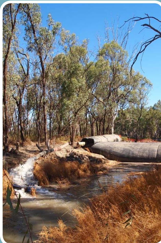
The Clark's Floodplain project used sandbags and an aquadam (inflatable dam, pictured above) to retain water in the target areas.
