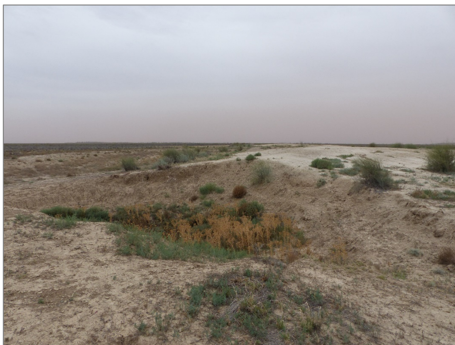
Figure 2-5 A breach in the western embankment on the lower western floodplain (photo: D. Ryder).
