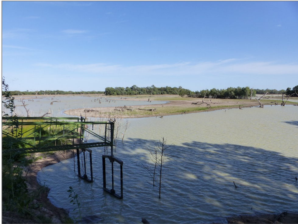
Figure 2-7 Boera Dam with regulator pipes in foreground, Western Floodplain bywash to the left and main Warrego river flowpath to the right (photo D.Ryder).
