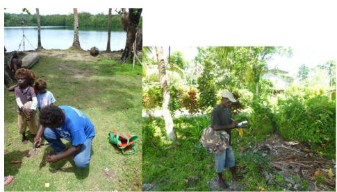
Figure 30 Marking contours with survey peg (left) and GPS (right)
