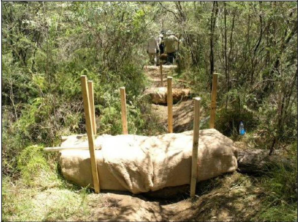
Figure 5.6 Small coir log dams (with jute wrapping) constructed at intervals along an incised swamp flow line.
