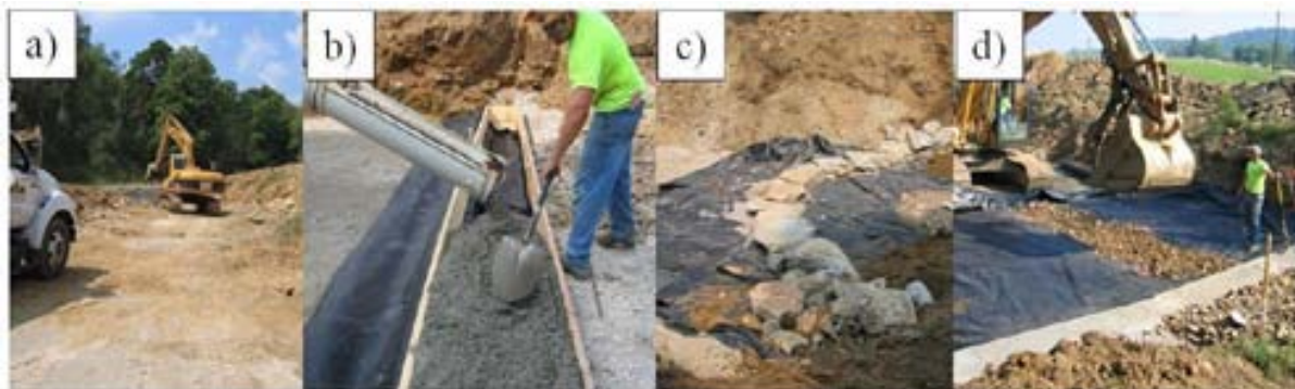
Figure 5.1 Geofabric installation to prevent water loss in streams with mining-induced tension fractures: a) stream-bed preparation; b) geofabric anchoring system; c) habitat controls; d) covering the geofabric.
