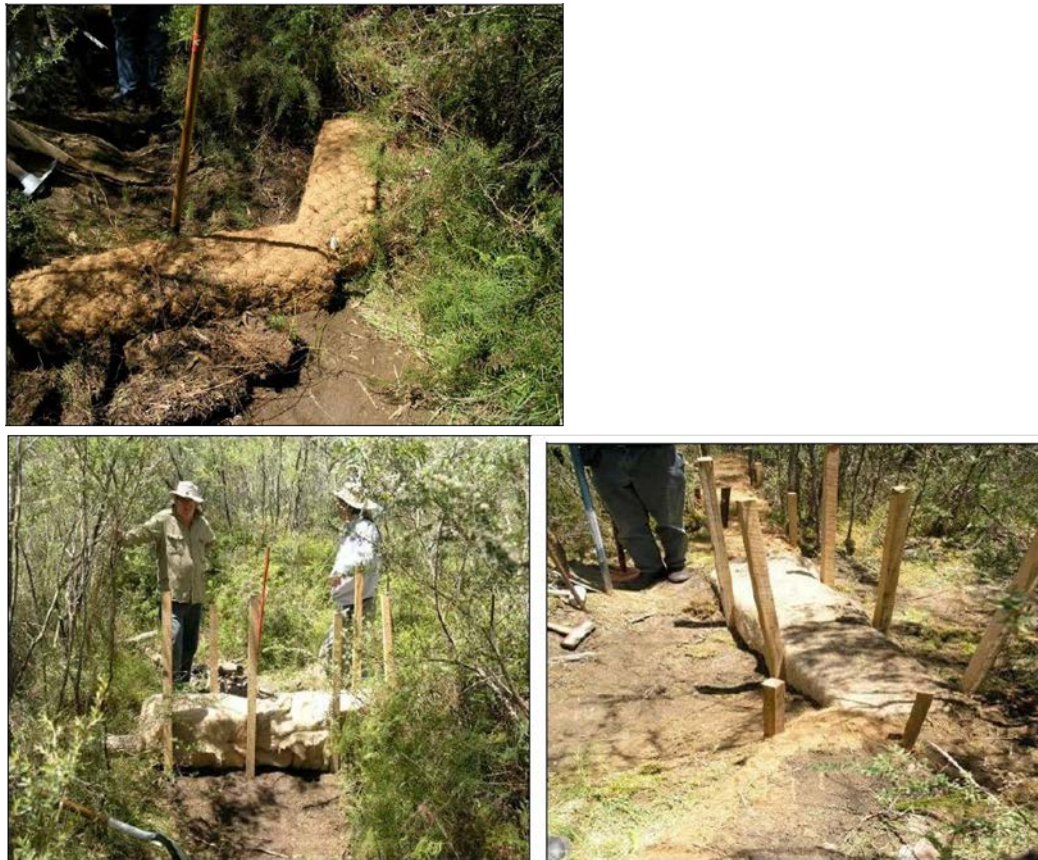
Figure 5.4 Square coir logs for knickpoint control.
