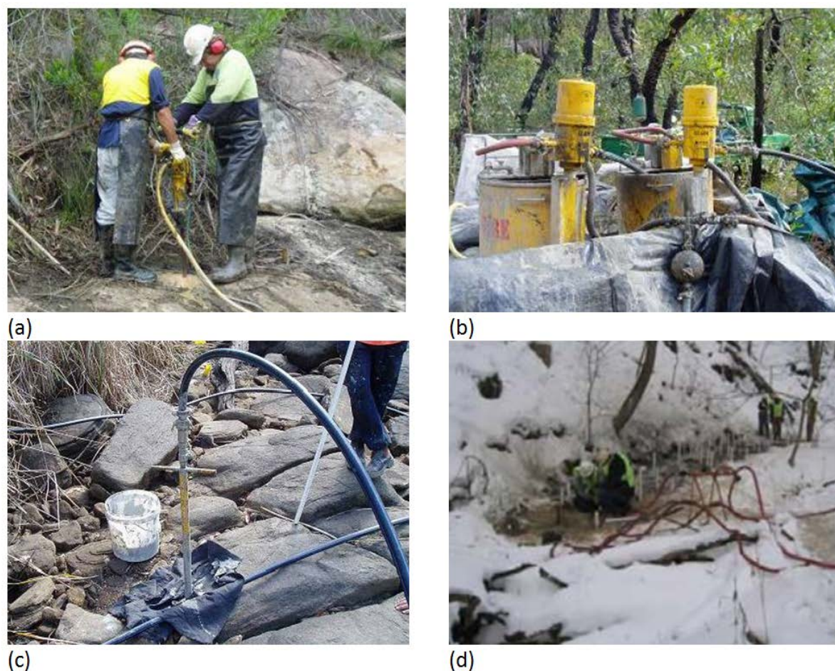
Figure 5.2 Injection grouting: (a) drilling into the bedrock (Georges River); (b) grout pump station set-up (Georges River); (c) injecting grout into the bedrock via packer system (Georges River); (d) grout injection operations (United States).
