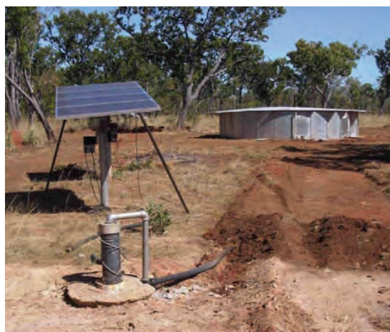
Figure 4.31 New waterpoint infrastructure on the Sturt Plateau
