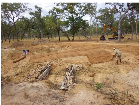
Balnggarrawarra Rangers undertaking gully remediation work on Normanby Station. Photos courtesy of South Cape York Catchments.
