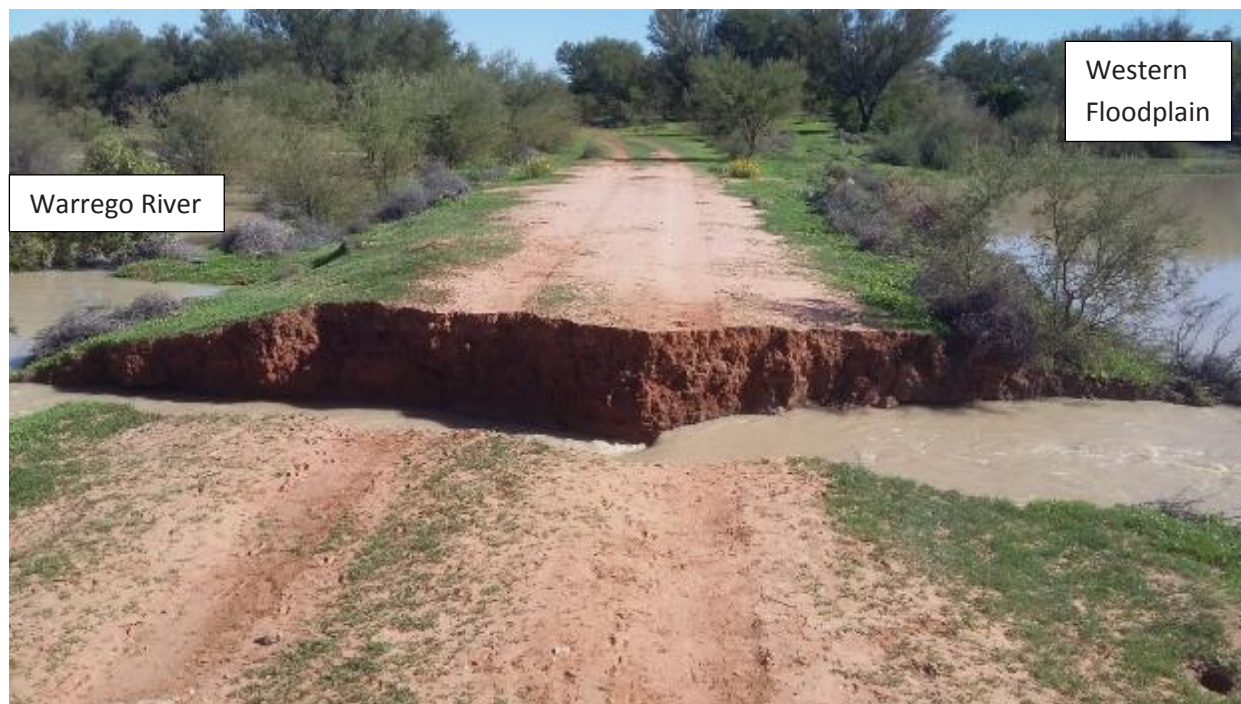
Figure E7: Breach in the eastern embankment between the Western Floodplain (right) and Warrego River (left)
