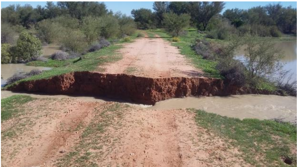
Figure 5: Breach in the eastern embankment between the Western Floodplain (right) and Warrego River (left)
