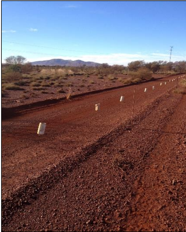
Figure 4 An early bat deflector design that was partially successful
