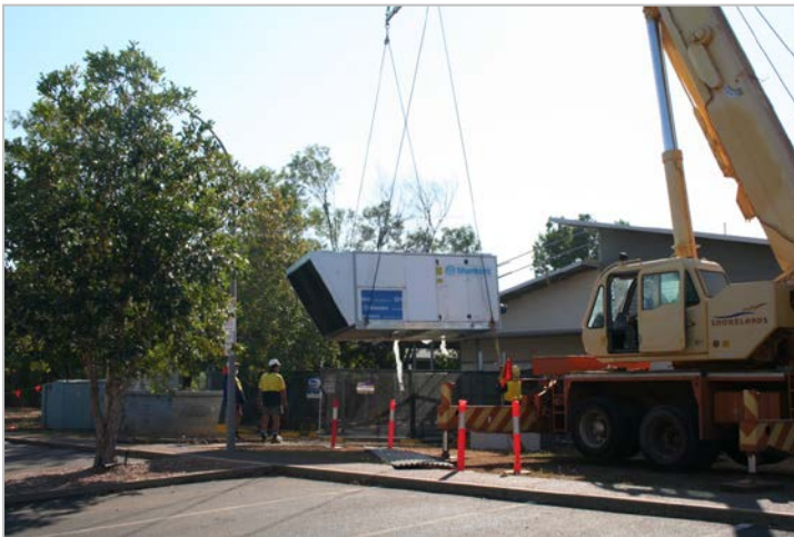
Figure 6.2 Dehumidification unit being lifted into position
