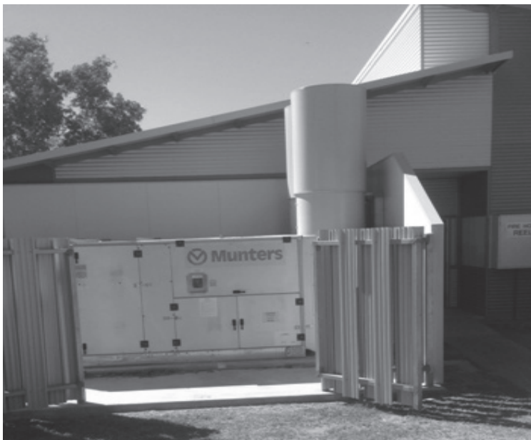
Figure 7.2 Dehumidification unit installed and functioning
