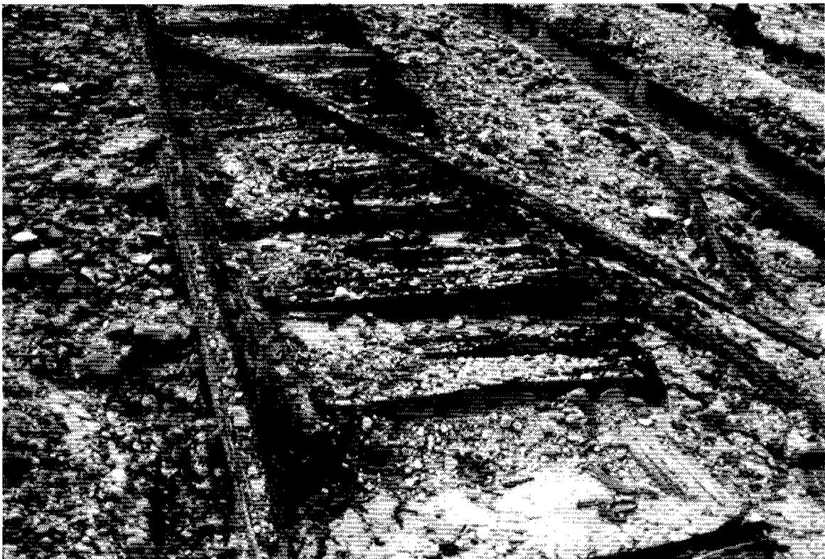
Plate 8 Deteriorating track-bed at Pyrite Wharf
