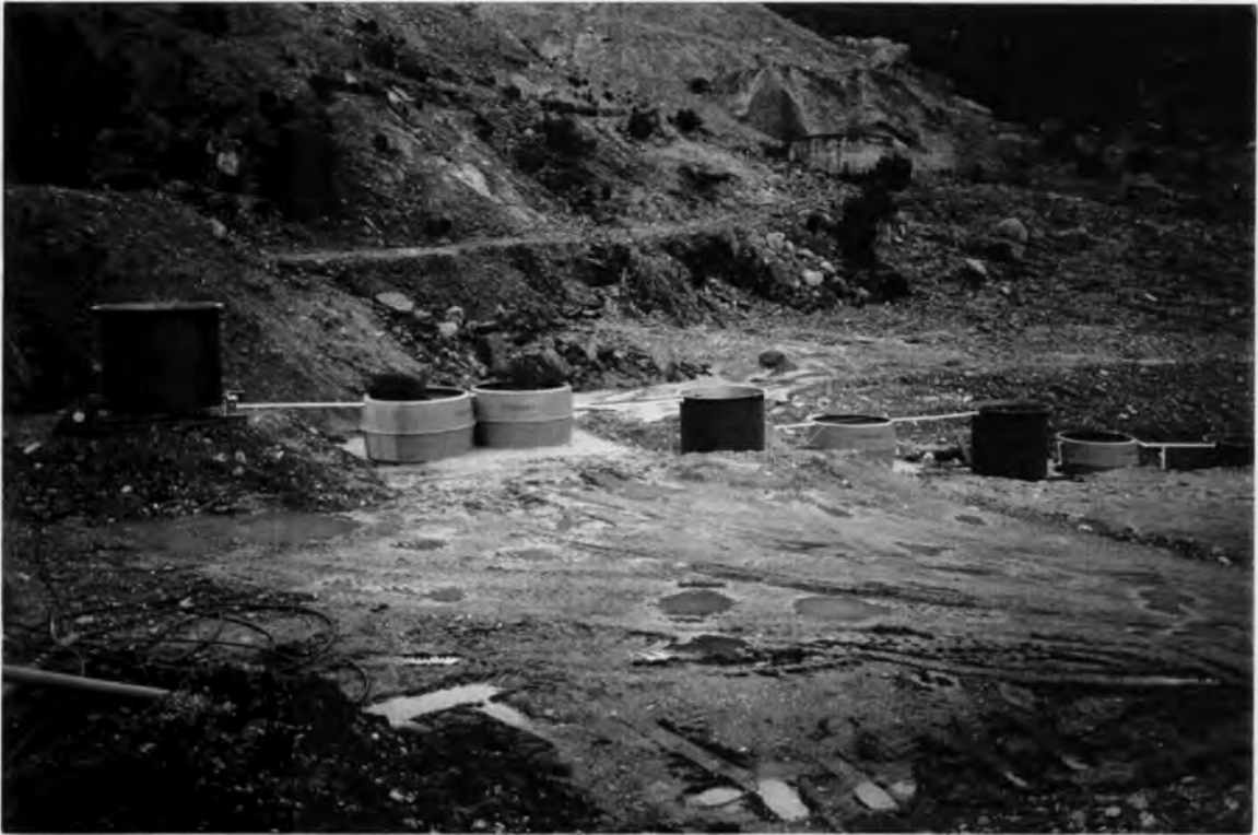
Plate 1 SAPS. Large black tanks are 'components' and smaller green tanks are 'marsh/settling' areas. Refer to schematic in figure 6.6.
