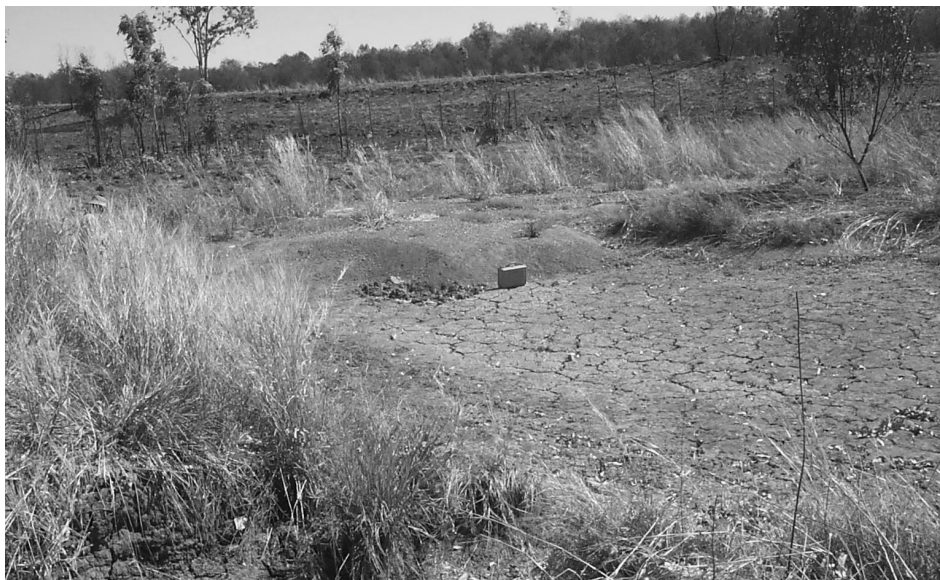
Plate 6 This is the sedimentation pond outside the south east corner of the boundary fence (Site 14). The breach is seen in the foreground. The bund wall at the southern end of the WRD can be seen at the top of the plate.
