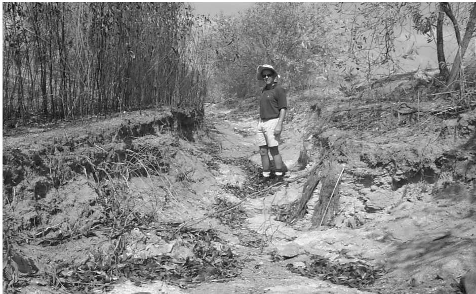
Plate 5 Incision in the base of the constructed earth drain parallel to the airstrip (Site 10)
