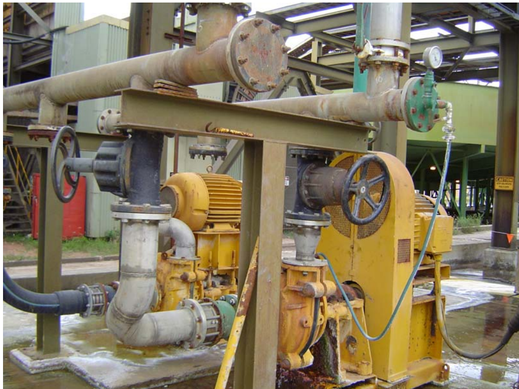
Booster Pumps – Faulty Valve shown on right Photograph 8
