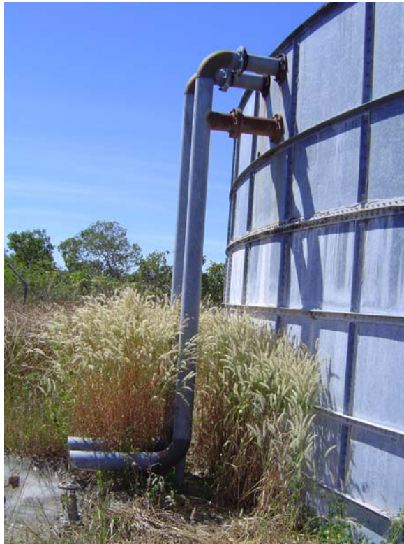
Booster Pumps – Faulty Valve shown on right Photograph 8
