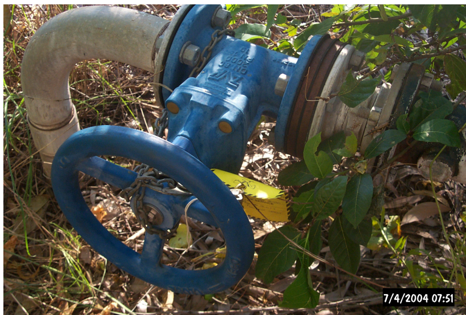
Figure 7 Jabiru Field Station main isolation valve
