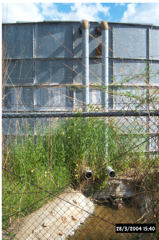
Figure 11 Jabiru East Potable Water Tank – overflow pipes and concrete drain
