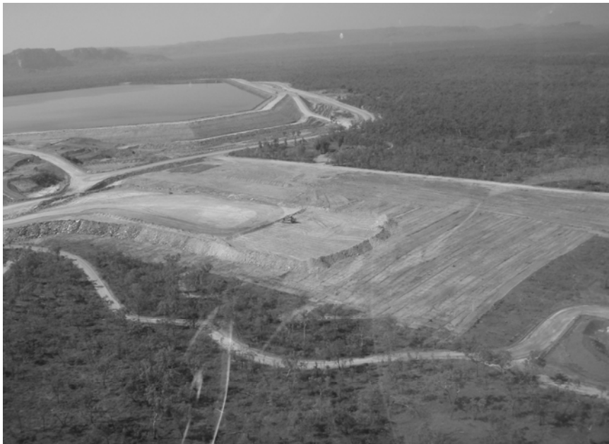
Figure 1 Trial landform prior under construction adjacent to the northwest wall of the tailings dam (20-Oct-08)
