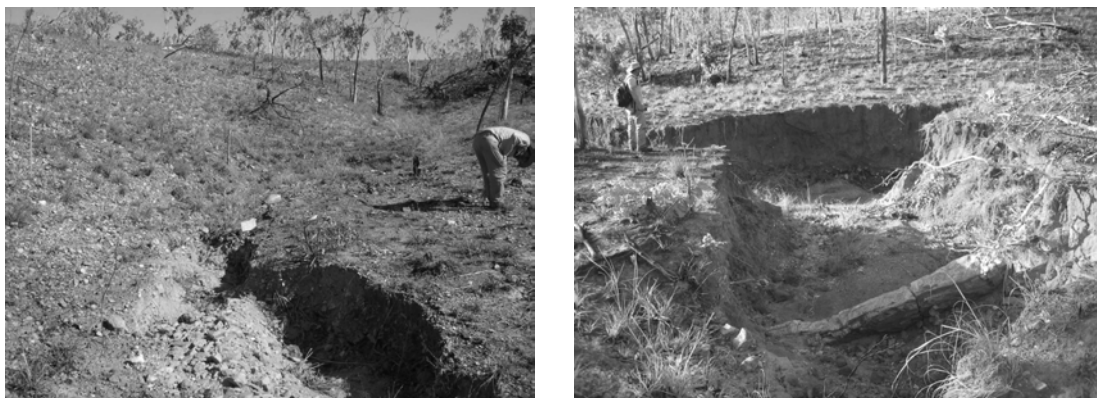
Figure 2 A medium (left) and large (right) size gully within the Tin Camp Creek catchment
