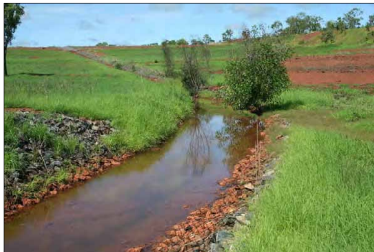
Figure 2 Accumulation of acidic and metalliferous runoff in subsided section of surface drain. Riprap seen in foreground of Fig 1 is upslope in this photo.
