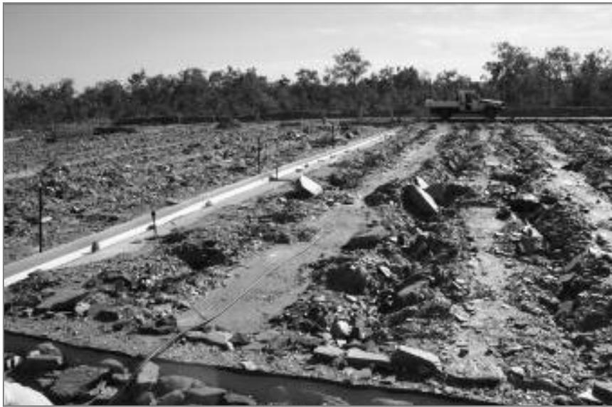
**Figure 3** Plastic half pipe trough and boundary
