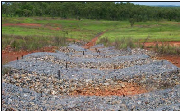
**Figure 1** Longitudinal drain in the cap of Dyson's Open Cut. Significant signs of subsidence can be seen in the vicinity of the single tree located towards the mid-background in the top right of the photograph. The drain has subsided here and acts as a basin to accumulate runoff. Signs of acid rock drainage are visible in the rock mulch in the bottom left of the photograph and in the drain toward top centre where rock mulch colour changes from grey to rust/brown.
