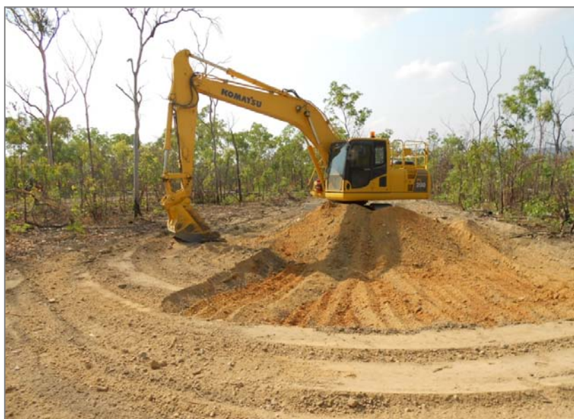
Figure 1 Mixing of the soil at one of the Magela B LAA rehabilitation plots
