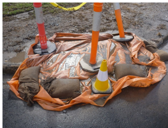
Figure 3.4 Example of drain blockage.
