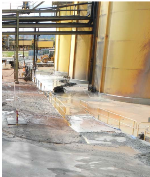
Figure 2.4 Leach tank bund following the failure of Leach Tank 1.
