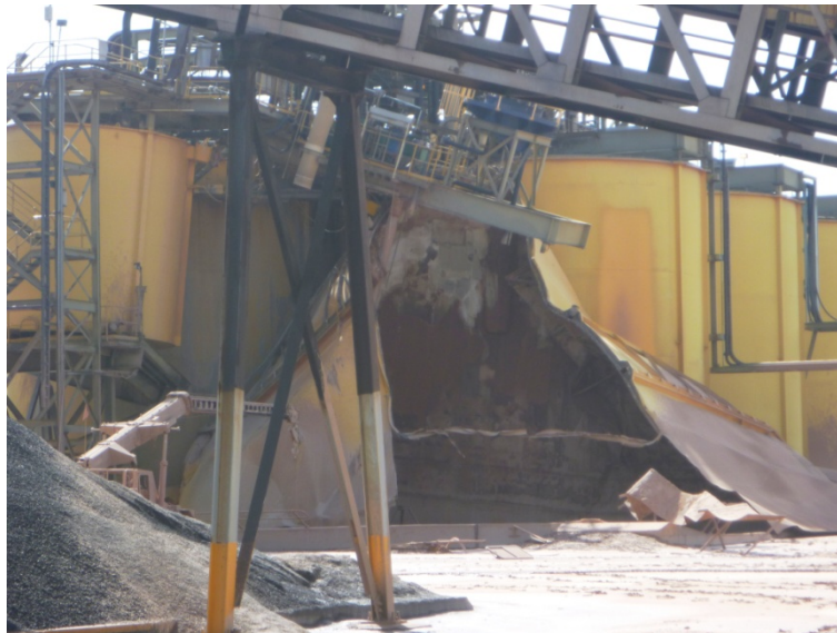
Figure 2.1 Collapsed Leach Tank 1.
