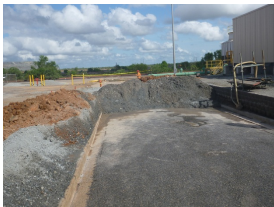
Figure 3.3 Containment bunding between RP2 & leach tanks.
