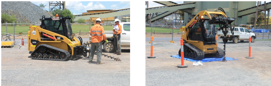
Figure 4.19 Auger mounted on a bobcat used to drill Hole 2.
