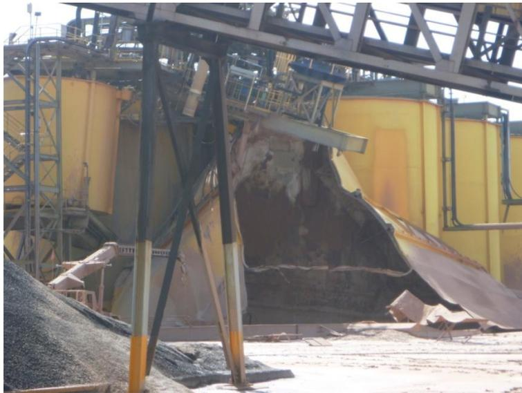
**Figure 2.1** Collapsed Leach Tank 1.
