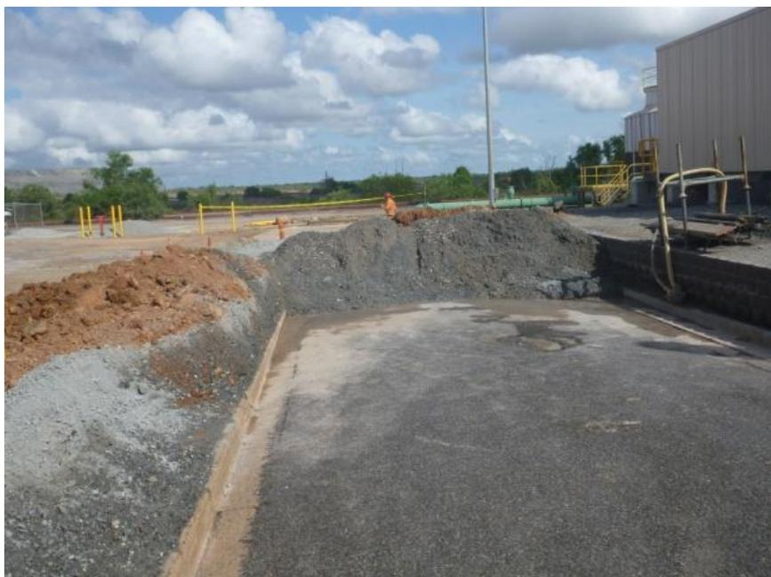
**Figure 3.3** Containment bunding between RP2 and leach tanks.
