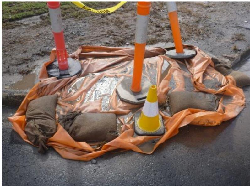
**Figure 3.5** Example of drain blockage.
