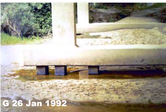
Figure 31 Hughes Creek at the old Hume Highway bridges at Avenel showing partial recovery of the sand slug since at least 1991. (A) and (B) Immediately upstream of Avenel stone bridge showing minor channel contraction between 1991 and 2014. (C), (D), (E) and (F) Avenel stone arch bridge showing the low flow channel and flood channel. (G) and (H) scour below the pile cap on the old Hume Highway bridge. Note that discharge is different between the two dates.
