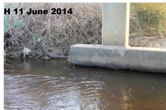
Figure 31 Hughes Creek at the old Hume Highway bridges at Avenel showing partial recovery of the sand slug since at least 1991. (A) and (B) Immediately upstream of Avenel stone bridge showing minor channel contraction between 1991 and 2014. (C), (D), (E) and (F) Avenel stone arch bridge showing the low flow channel and flood channel. (G) and (H) scour below the pile cap on the old Hume Highway bridge. Note that discharge is different between the two dates.
