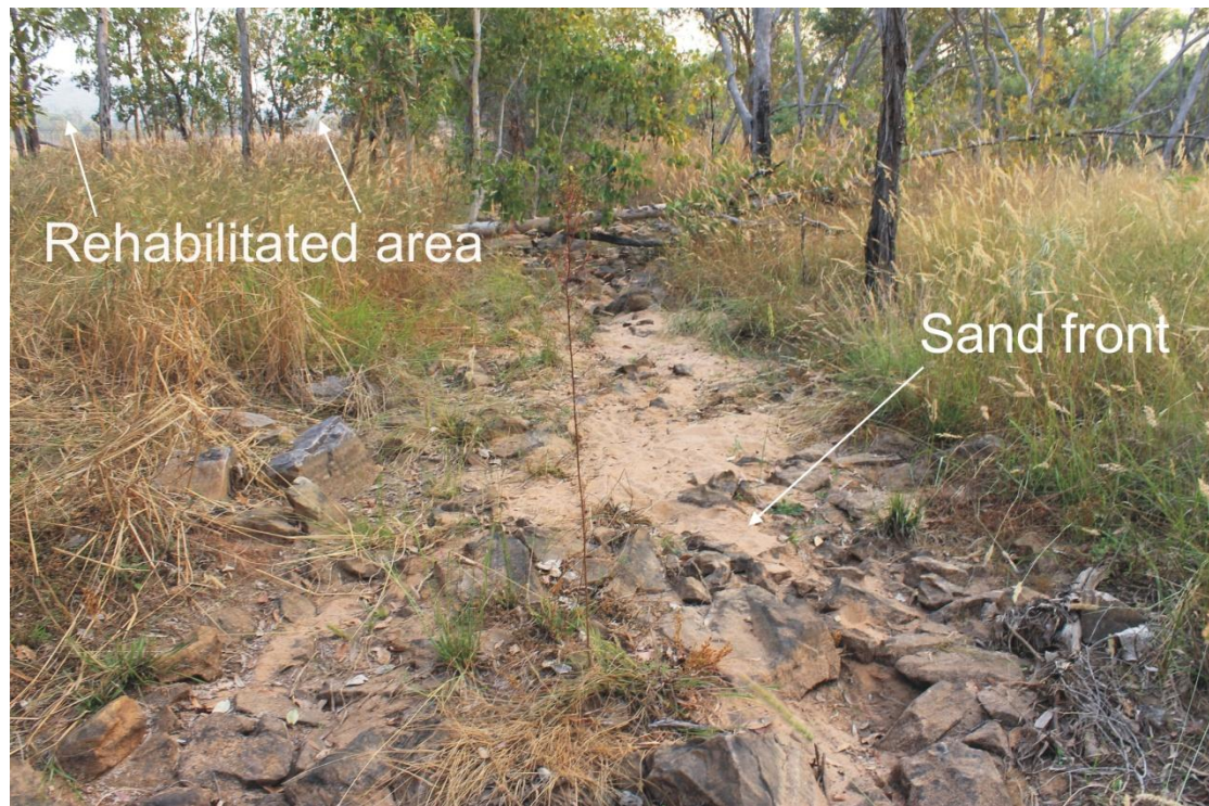
Figure 13 Tributary North looking upstream at the front of the sand slug. The open spaces of the rehabilitated area can be seen through trees at the top left of the image. Image taken 17-7-14.
