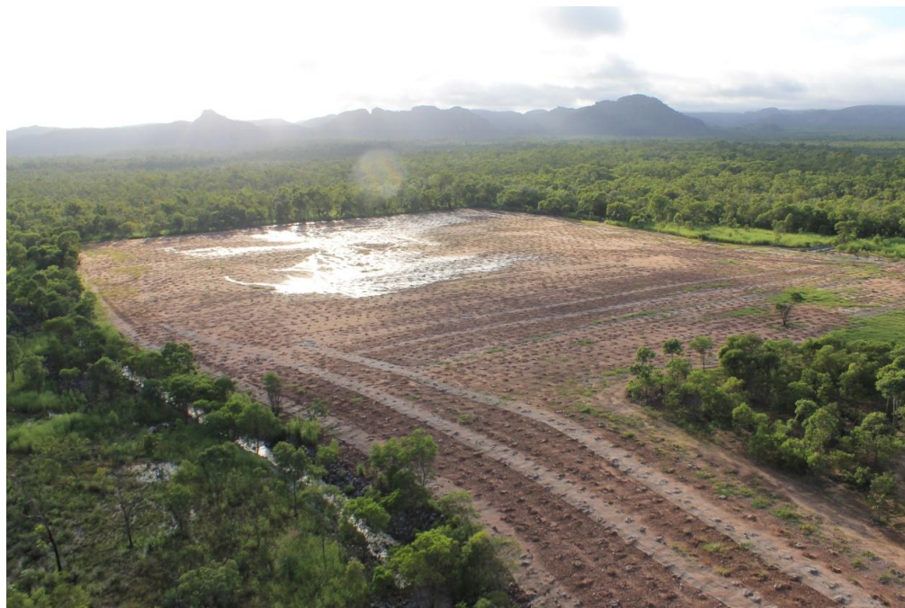
Figure 1 Aerial view looking east over the rehabilitated IWMP. Water on the lower half of the slopes suggest a seep where water is coming out of the ground. Image taken 20-2-2014.
