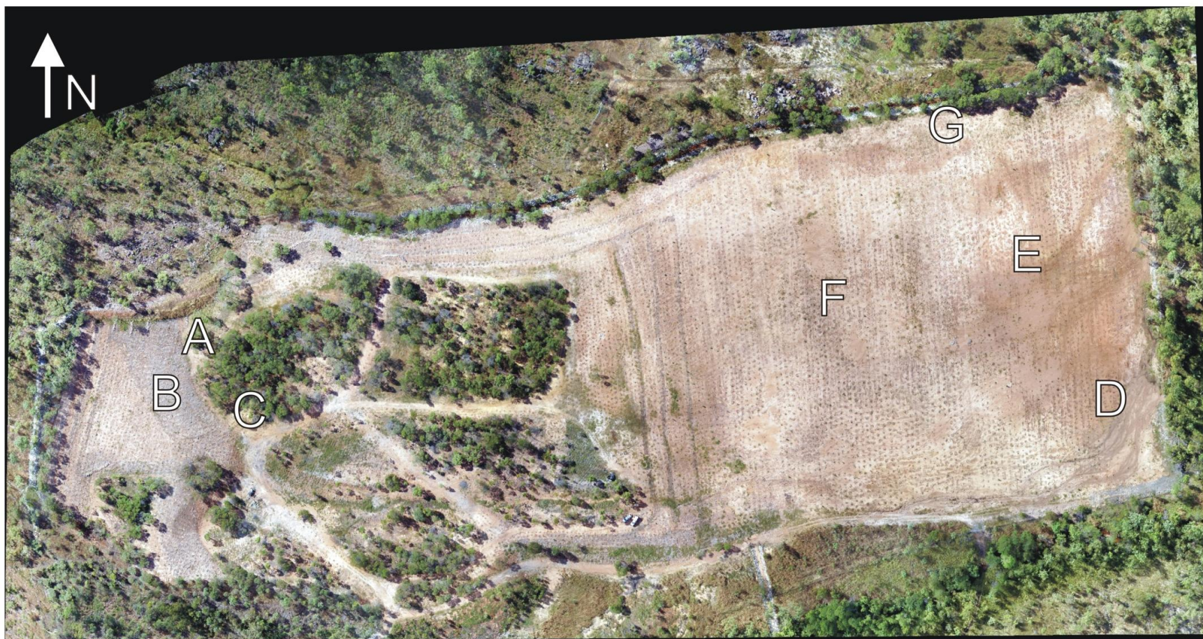
Figure 2 Jabiluka mine site April 2014. Letters refer to photo locations in the document.
