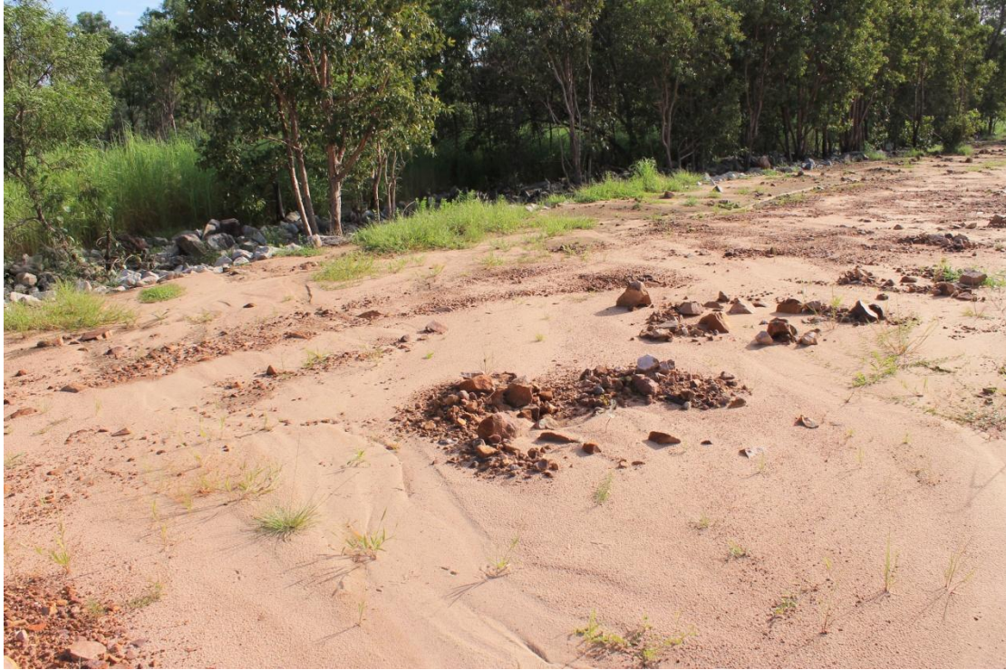
Figure 9 Sand deposited on the area just upslope of the bank of Tributary North at Site G on Figure 2. Image taken 20-2-2014.
