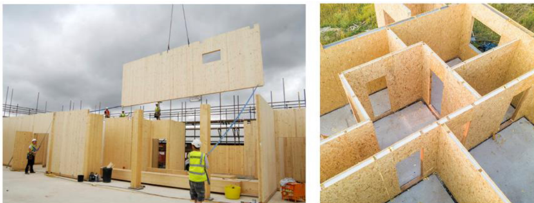
Figure 38 – Assembly of prefabricated mass-timber
