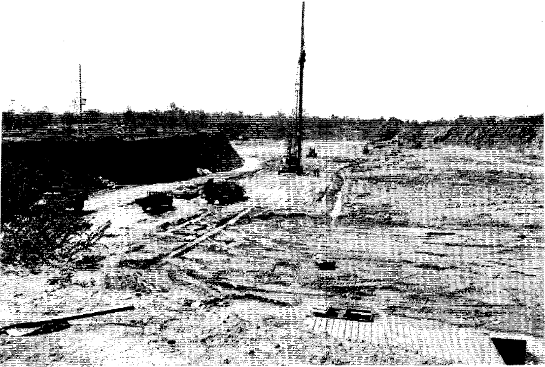
Plate 4. Placement of geotextile and waste rock cover: Dry season 1988
