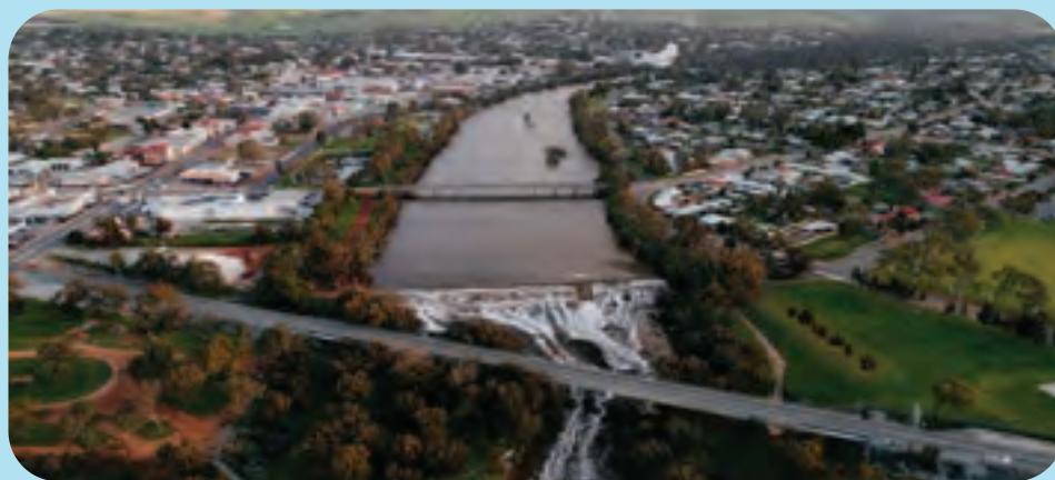
Image courtesy: Shire of Northam
