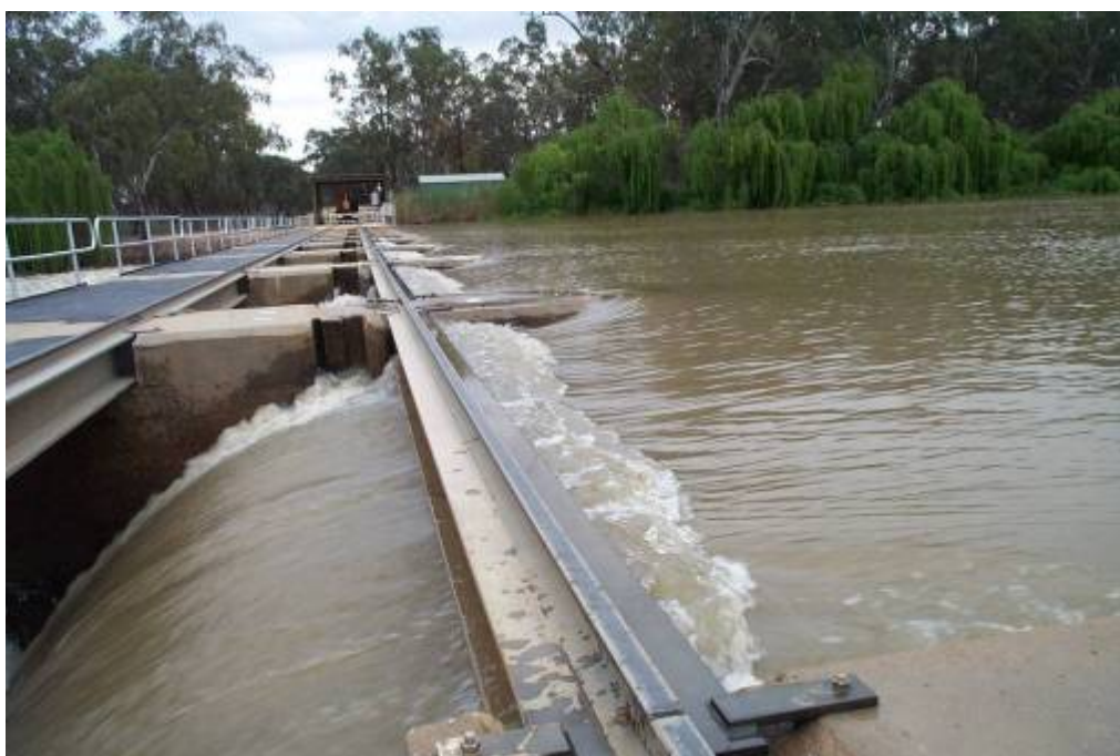
Weir pool raising at Lock 5 - normally about 50 cm below this level (Source: Tony Herbert, CSIRO).
