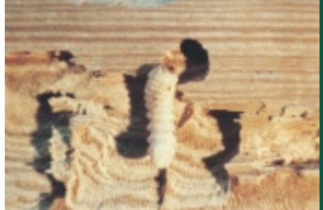
Damage caused by European house borer larva
