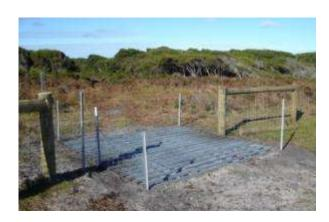
Figure 2 Installed wallaby grid on King Island.
